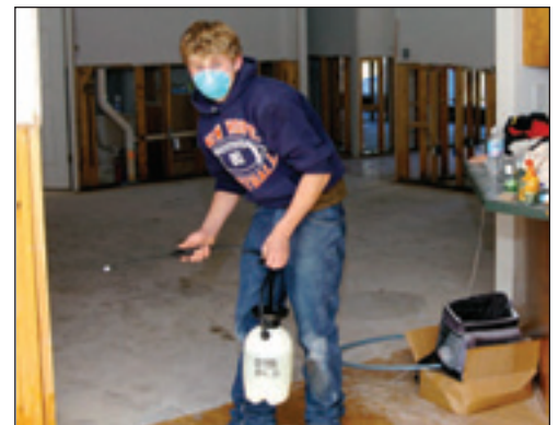
Justin Harris sprays a bleach mixture to kill mold.
